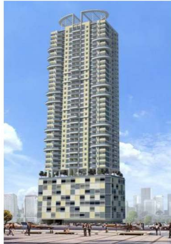
Wharton Parksuites - Manila 40-story building
